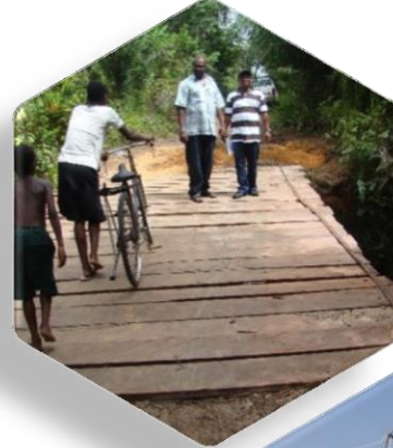
Bridge was constructed in Imiringi Community, Delta State.
