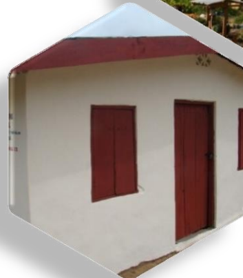
Renovation of Town hall for Adagbabiri community
