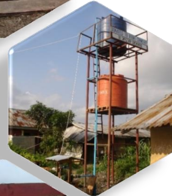
Drilled Water well for Ofoni Community in Bayelsa State
